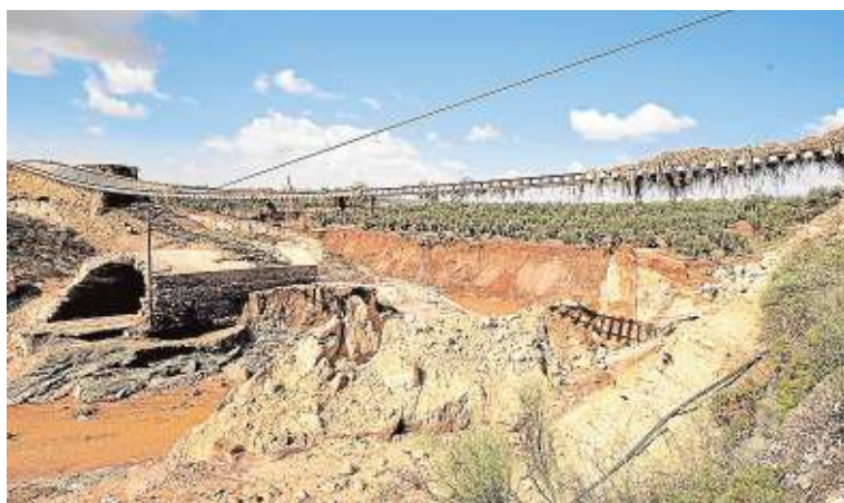
The condition of the railway track after the flooding. :: NITO SALAS
