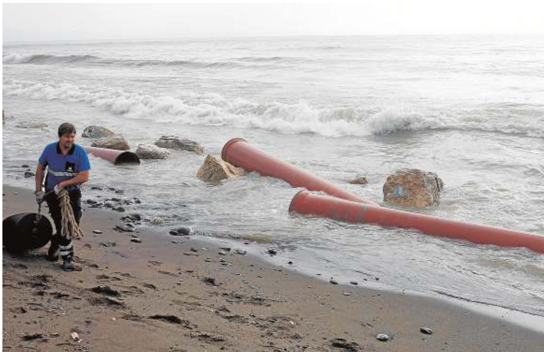
The main sewage pipe under San Pedro beach was broken this week by the strong waves. ■ JOSELE-LANZA
