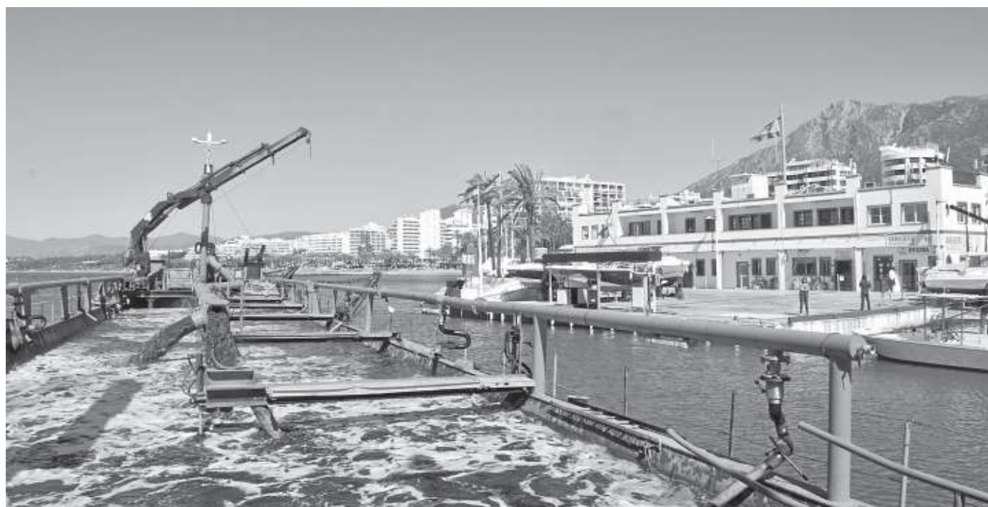
The sand is taken from four metres of water at the mouth of the leisure marina and discharged into the hold. :: JOSELE-LANZA
