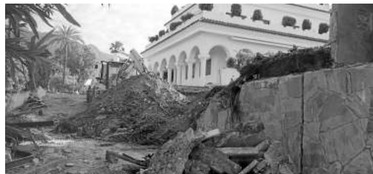
Demolition works on the wall which was at risk of collapse. ■ SUR
