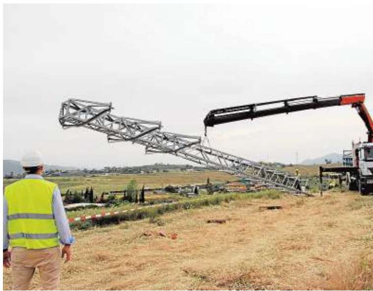
One of the first power pylons being erected. :: SUR
