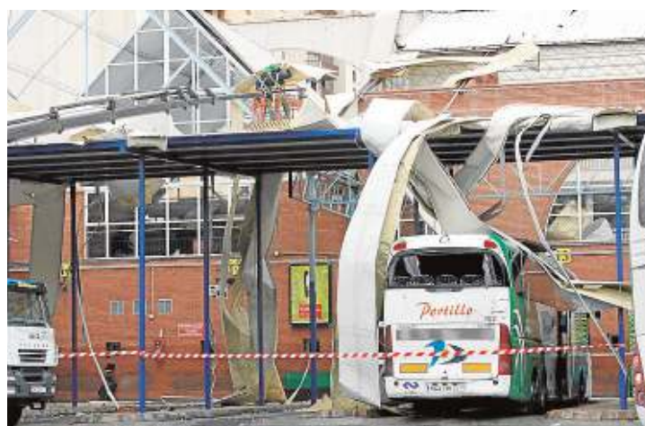
Extensive damage to the bus station roof. :: CARLOS MORET
