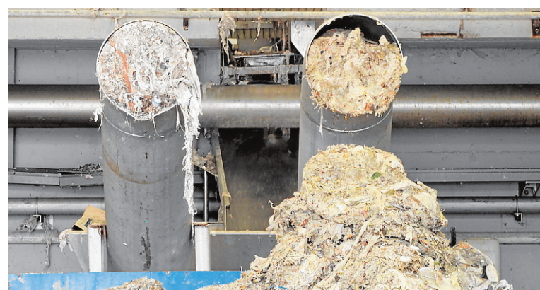
Sewage pipes blocked up with wet wipes. SUR
