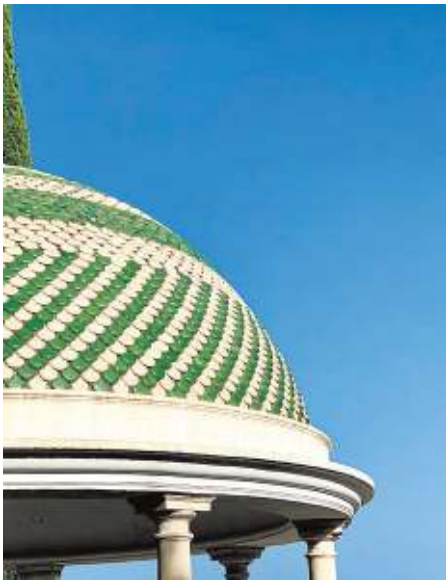
La Concepción Botanical Garden. The cupola built in 1920 and located on the southern hill of the garden has a roof made of green and white scale-shaped glazed tiles. SUR
